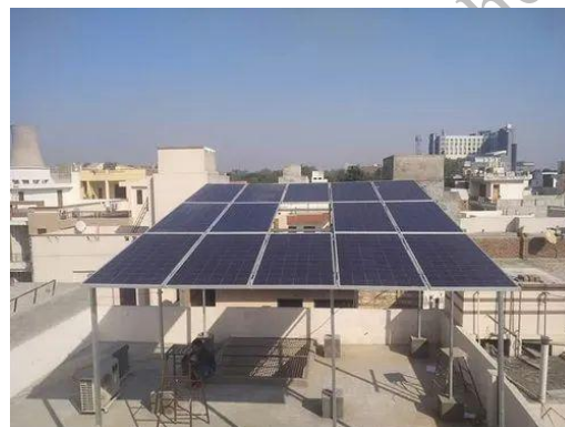
Fig. 4.10 Rooftop Mounted Solar PV System
