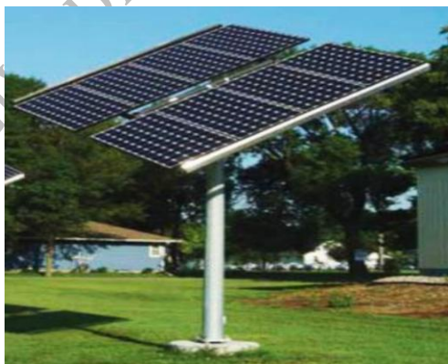
Fig. 2.24 Single Pole Mounting Solar PV Structure
