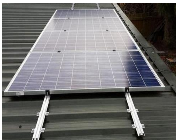
Fig. 3.20 Railed Mounting System
