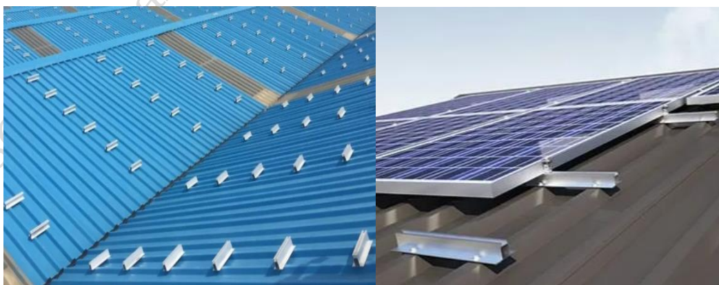
Fig. 3.24 Tin Shed Mounting Structur
