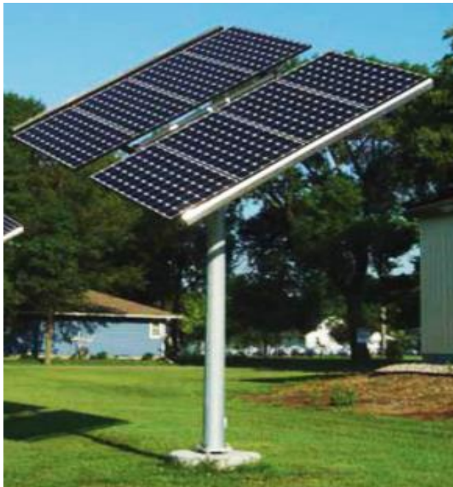
Fig. 3.27 Pole Mounting Structure
