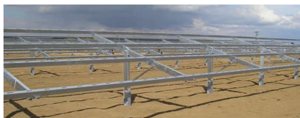
Fig. 3.25 Foundation Mounting Structure
