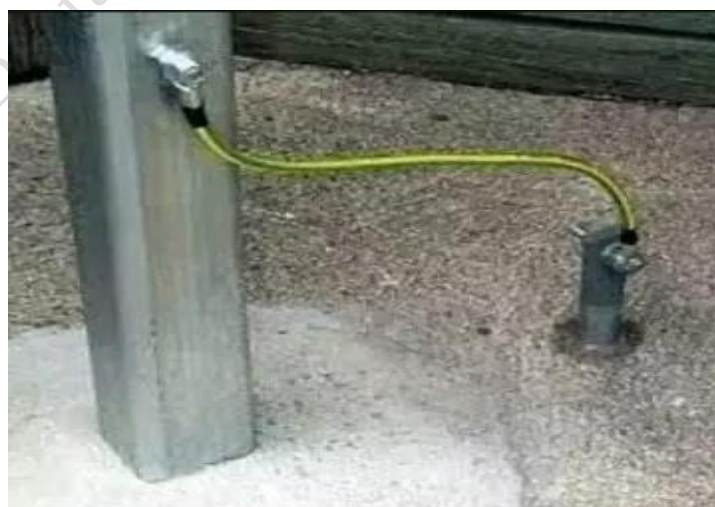
Fig. 3.45 Pipe Earthing
