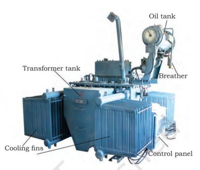
Fig. 1.21: Transformer parts
