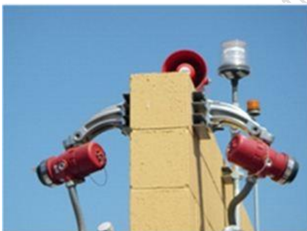
Fig. 4.11: Flame Detection Systems
