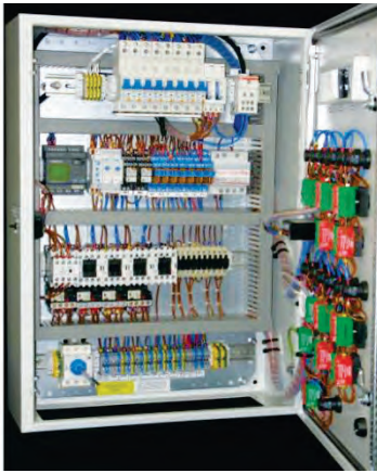
Fig. 8.16(a) Correct raceway (routing) of cable
