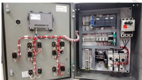
Fig. 8.12 One-door control panel
