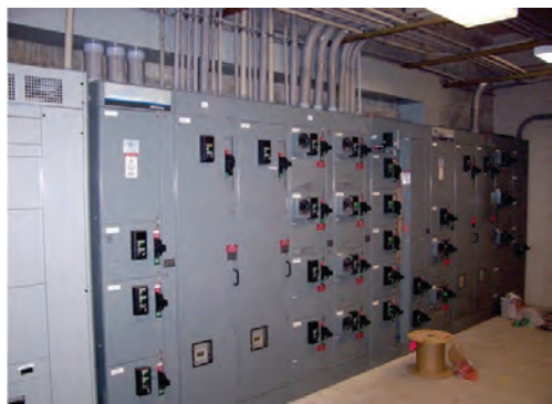
Fig.8.10 Motor control centre in control panel
