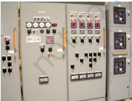
Fig. 8.8 Switch gear cabinet in control panel
