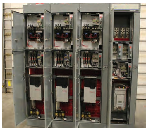
Fig. 8.11 MCC bucket centre assembly in control panel
