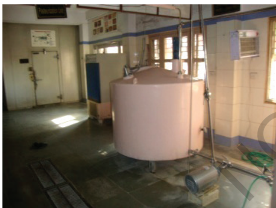
Fig. 4.12: Refrigeration facility at a bulk milk room in a farm
