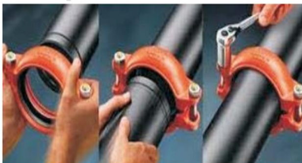
Fig 5.25 Grooved Joints
