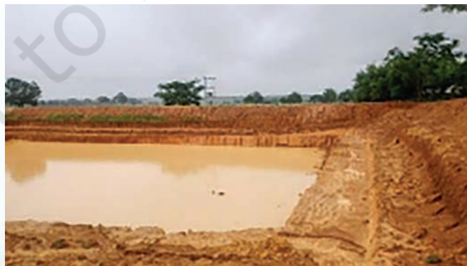
Figure 5.13: Percolation tank for groundwater recharge
